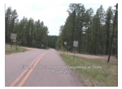
Beginning at SR 260 the existing paved portion of the road will have centerline and edgeline rumble strips added. The next 1.75 miles of gravel road will be a double chip seal (24' wide).
