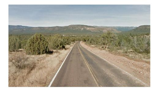
Add 5' wide paved shoulders, install centerline and shoulder rumble strips. Add curve warning signs.
