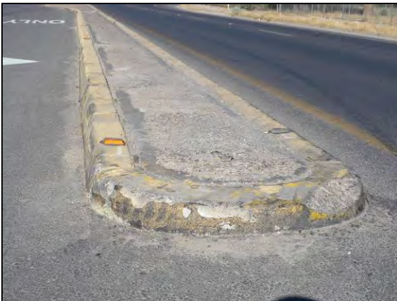
Figure 14: Missing RPMs and Faded Paint Make It Difficult to See the Median Bullnose at Night
