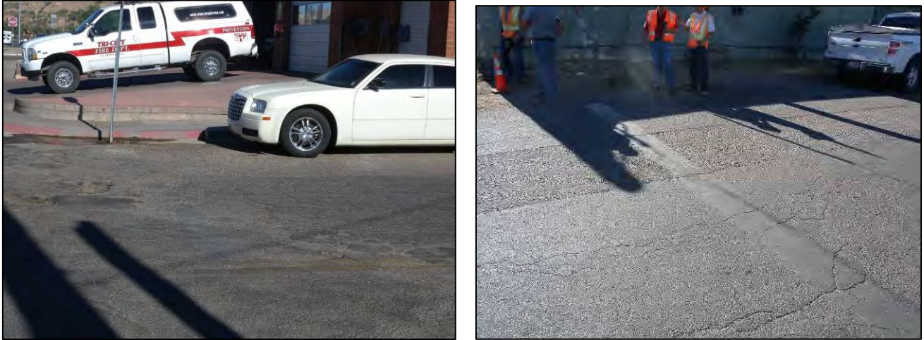
Figure 15: Faded Centerlines and Stop Bars
